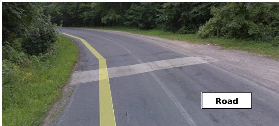
Fig. 1. Road fault causing a loss of stability
